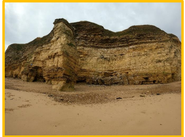
Caves and arches along toe of cliffs adjacent to Wife Lot (/0401C03)
