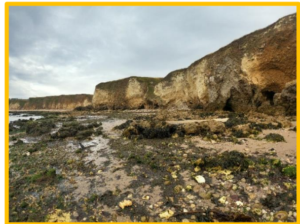
Rockfall at northern end of Marsden Bay (/0401C04)
