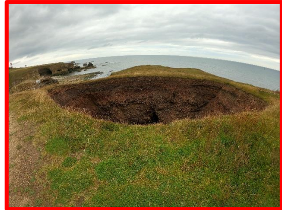
Enlarged sink hole at the former Old Harbour Quarry (/0501C01)
