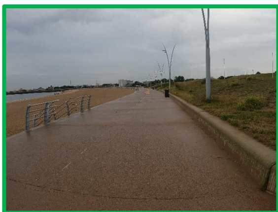
Littlehaven promenade and seawall in very good condition (/0102C02)
