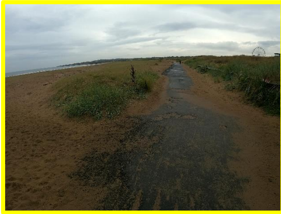
Southern section of the 'donkey track' showing surface deterioration (/0201C01)
