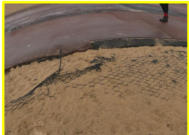
Previously buried rock mattresses exposed in 2022 (/0202C01)
