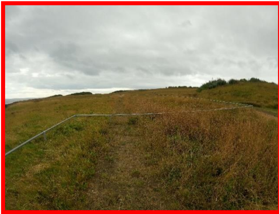
Fencing to divert the public around a new sink hole at Whitburn Coastal Park (/0501C01)
