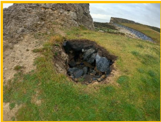
Reopened sinkhole landward of Target Rock (/0302C03)
