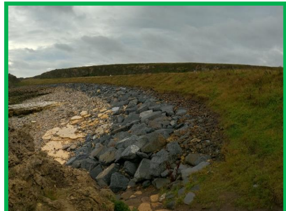
Rock revetment and re-graded slope at Southern Bay (/0302C04)
