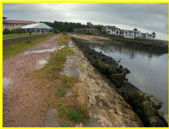
Grouted masonry revetment in fair condition (/0101C01)
