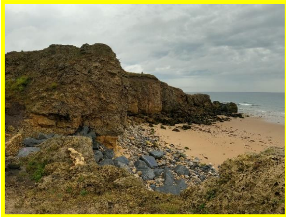
Southern aspect of Trow Point (/0302C01)
