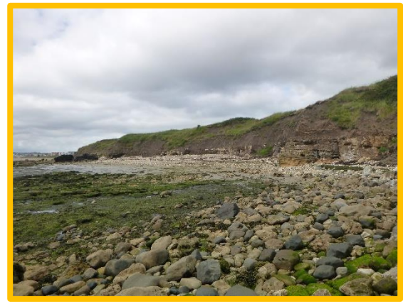
Thin limestone cliff mantled with thick glacial till layer. Generally, more active than cliffs to the north. (/0601C01)
