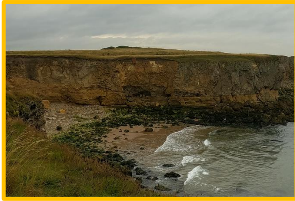
Undercutting at base of cliffs at Frenchman's Point (/0401C04)
