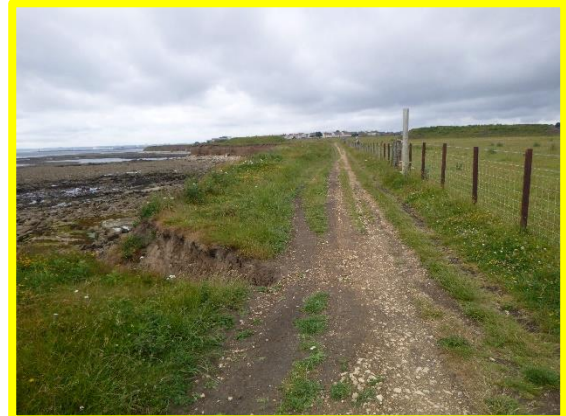
Surface water local scouring back the softer glacial till layer. (/0601C02)
