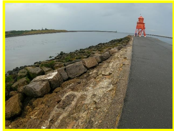
Additional armour stones placed on river-facing side of South Groyne (/0101C02)
